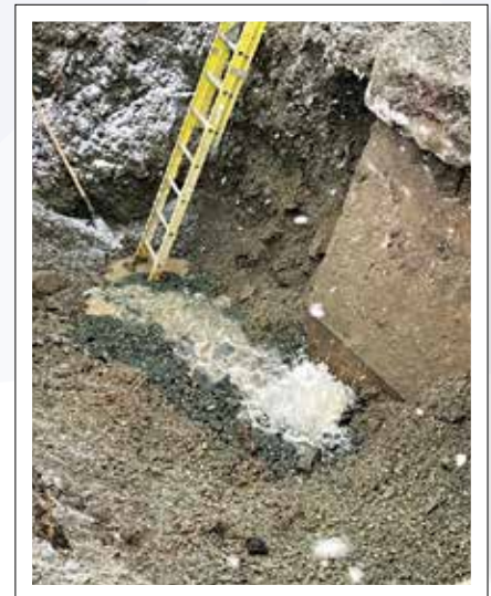
Leaking watermain before water was shut off.
