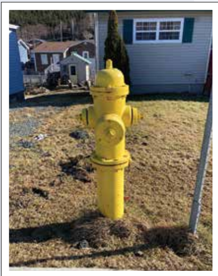
Typical photo of a fire hydrant with a leak detection sensor in the pumper cap.
