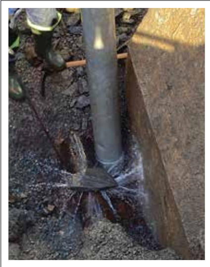
Leaking watermain after water was shut off.
