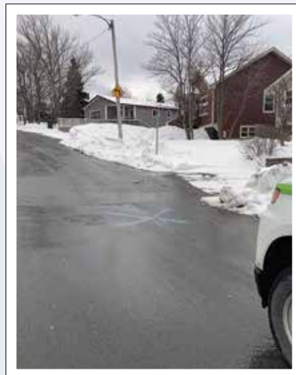
Location of watermain leak detected by the leak monitoring system.
